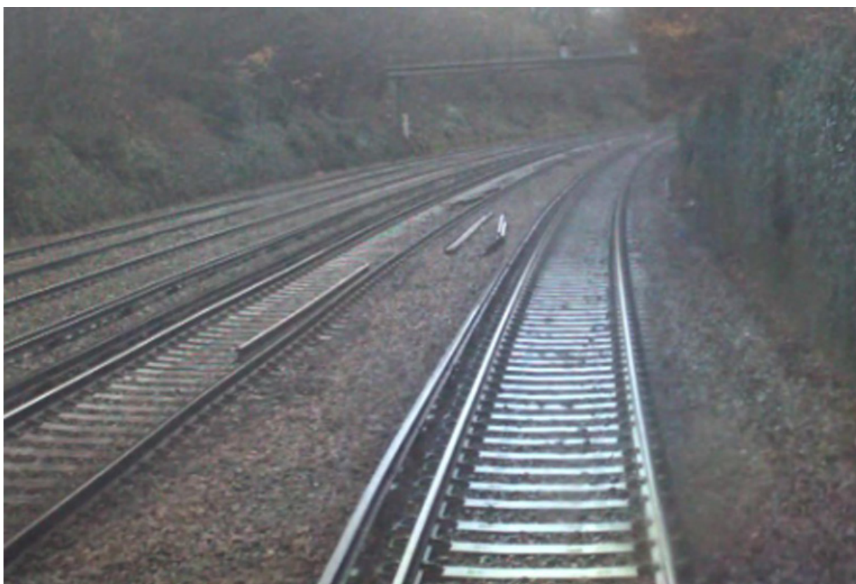
Figure 15: Photo of the FFCCTV from the inspection train used in the email from the project lead to other Colas Rail staff as an 'example of the scrap rail, present in 6ft and adjacent road' (courtesy of Network Rail).
