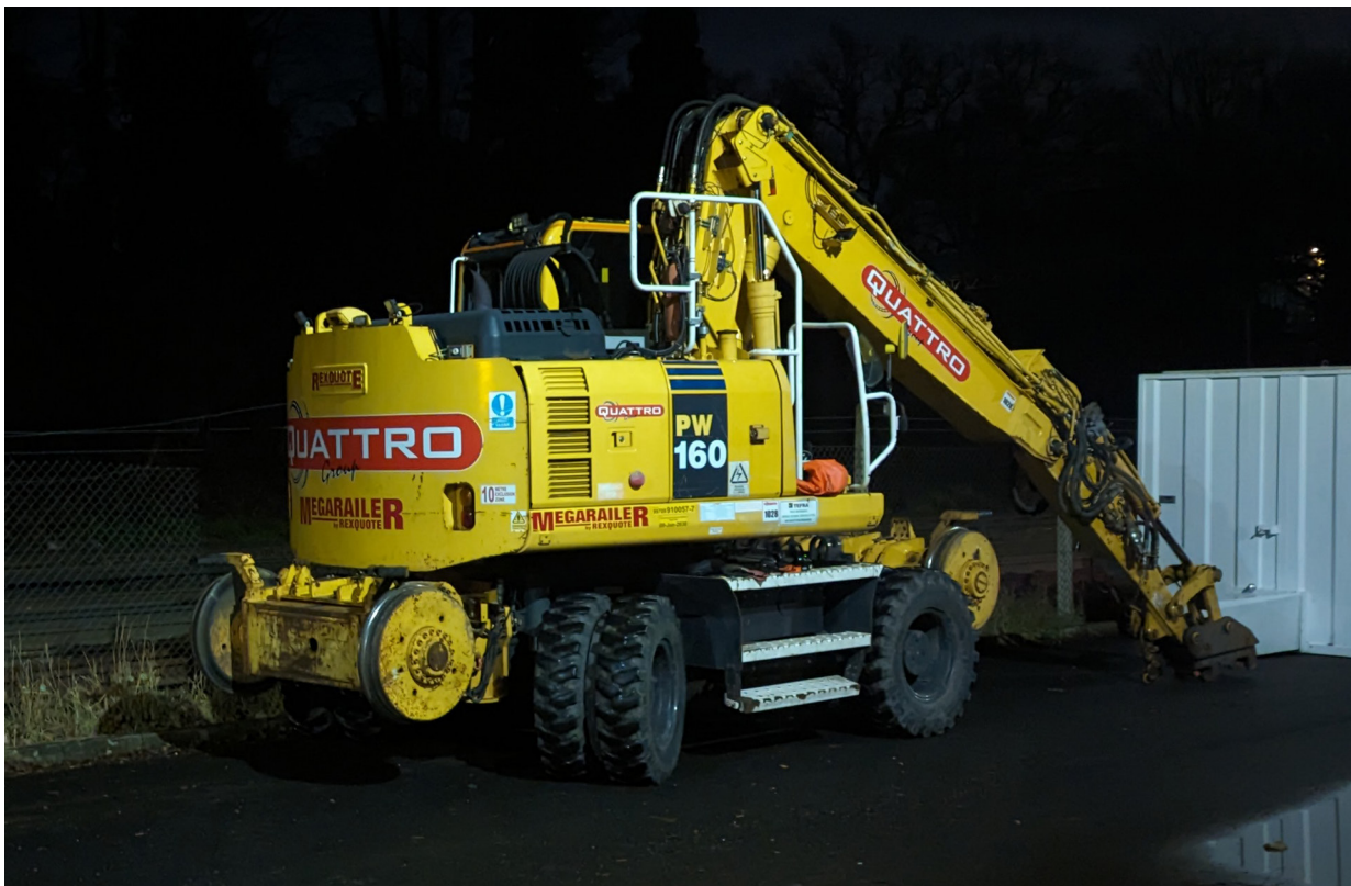
Figure 4: RRV used at the work site near Walton-on-Thames.
