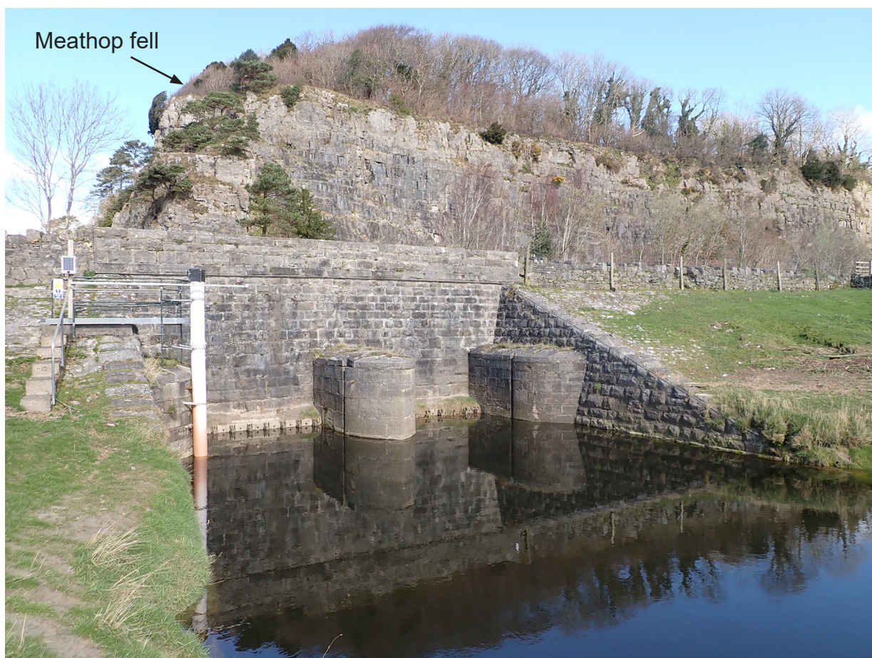
Figure 7: Tidal gates on the River Winster.
