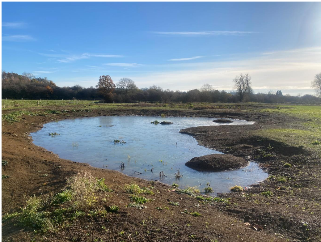
Figure 15 - Cottesbrooke offline storage area (image credit: Ryan Jennings, JBA Consulting)
