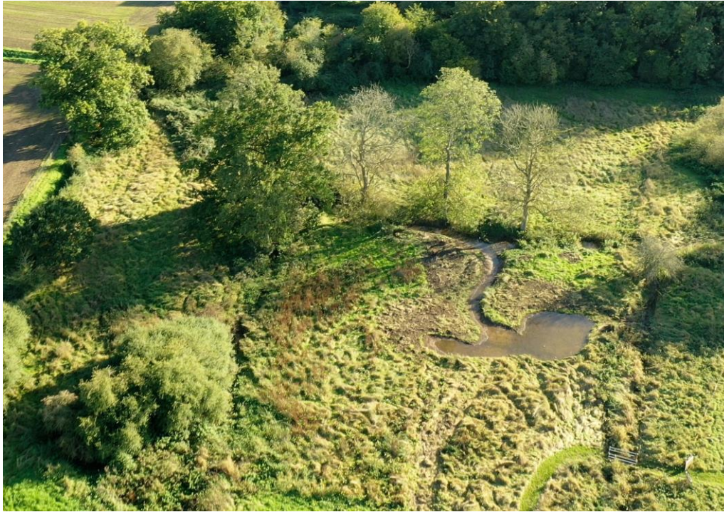
Figure 8 - Floodplain attenuation wetland, Gissing (image credit: Norfolk Rivers Trust)
