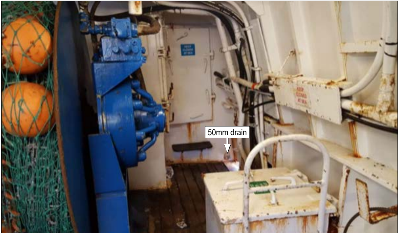
Figure 6: Position of the drain from the starboard passageway
