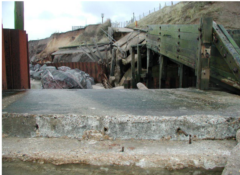
Figure 9.2 Close up of Happisburgh defences
