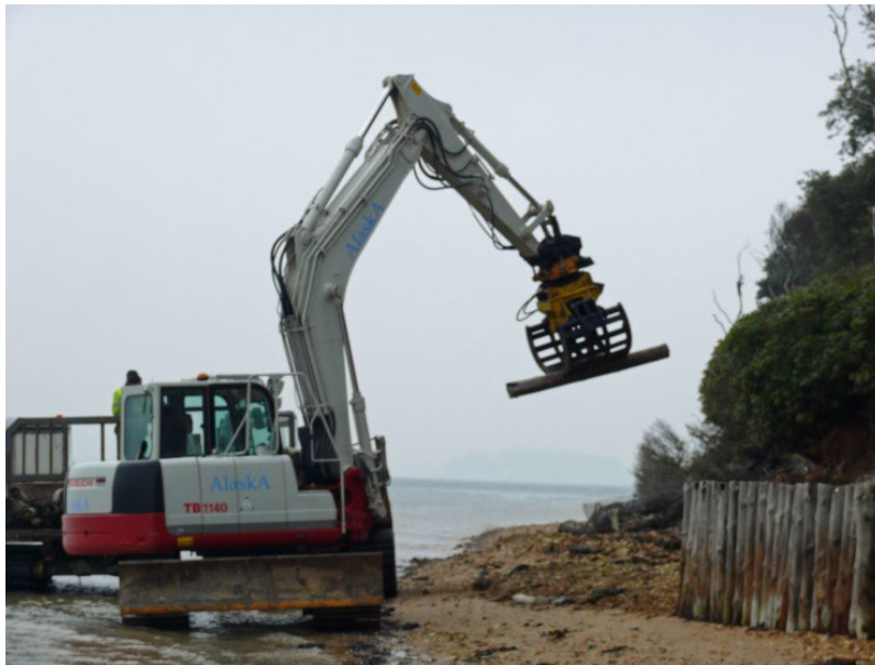
Figure 9.4 Brownsea site during decommissioning works
