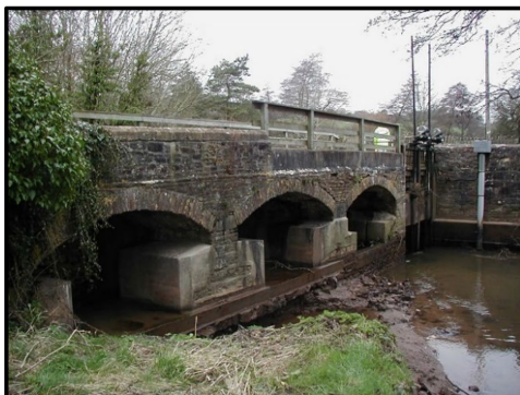
Bridge with sluices
