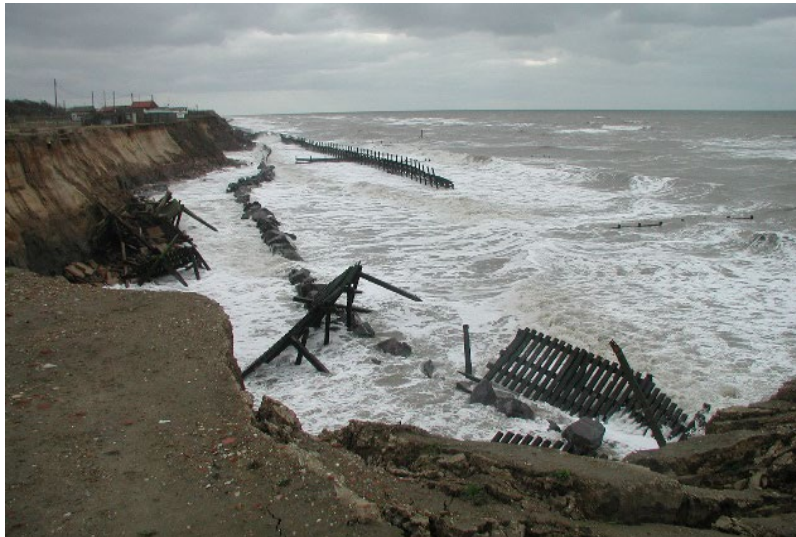
Figure 9.1 Failed Happisburgh defences
