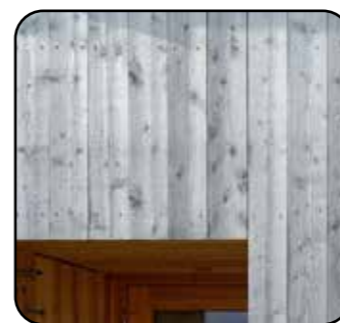
6" vertical timber - silver Face-fixed, knotted character minimally spaced joints
