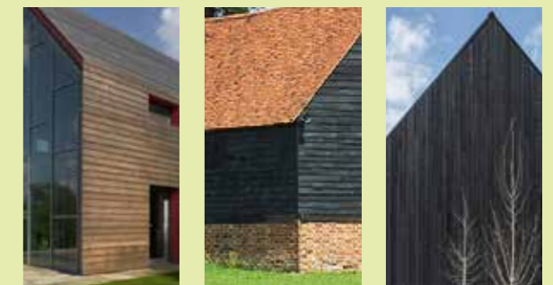
Glazed gable ends with timber cladding Traditional mix of materials - base, siding, roof Vertical timber rainscreen cladding - dark, natural, light
