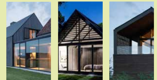
Glazed linking elements connect larger massing volumes Recessed south-facing windows with brise soleil for shading Recessed south-facing windows with screening on overhang
