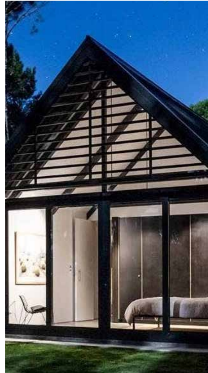
Recessed south-facing windows with brise soleil for shading
