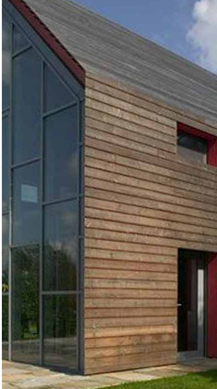
Glazed gable ends with timber cladding
