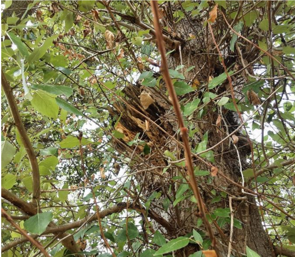
Photograph 3: Tree 2, poplar. Cavities located in the tree trunk.
