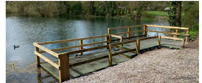
The completed restoration of the banks of Hampden Pond.
