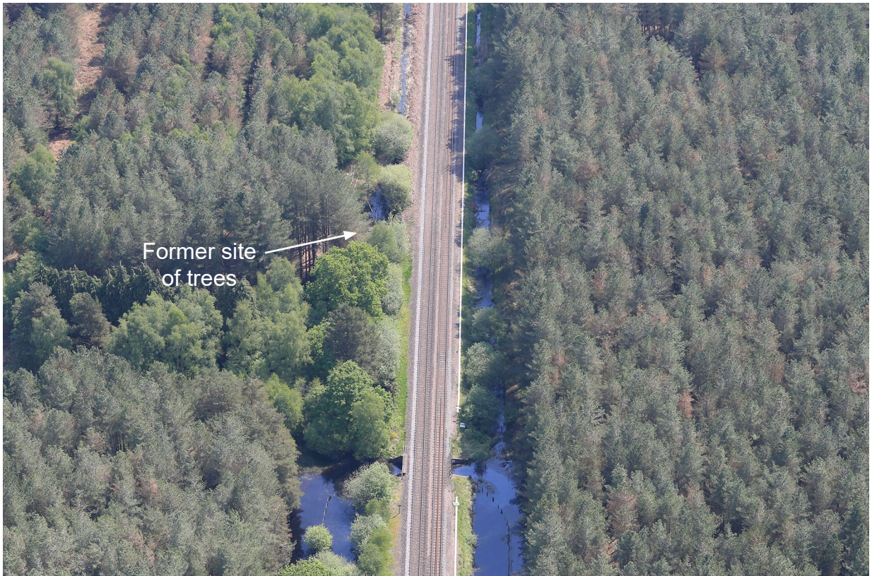
Figure 7: The extent of flooding at the site in May 2024, just over 3 months after the accident. The previous location of the pine and oak trees is indicated (courtesy of Network Rail, with RAIB annotations).
