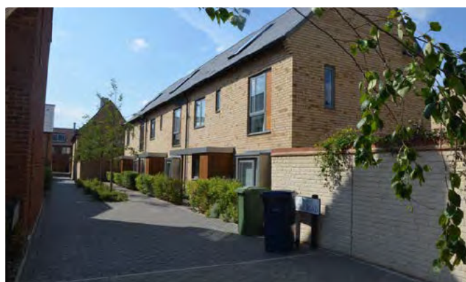
▲ Homes along narrower living streets in Trumpington Meadows are oriented to ensure maximum opportunity for ventilation and natural light.
