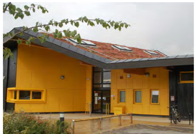
▲ Green roof in Broughton, Milton Keynes is an effective strategy to reduce surface runoff and recycle rainwater.
