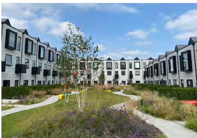
▲ Modular housing provides a resource-efficient method of construction in Port Loop, Birmingham.
