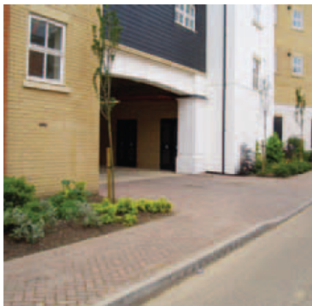
Undercroft secure parking (gated entry).
