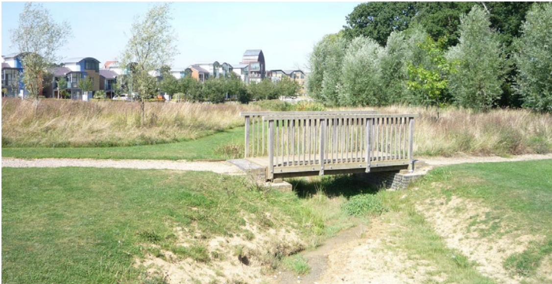
Sustainable drainage at the New Hall development in Harlow, Essex
