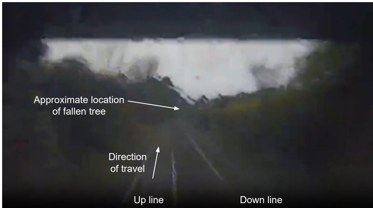
Figure 19: Image taken from train 1A37 forward-facing CCTV as it passed under the road bridge (courtesy of ScotRail with RAIB annotations).
