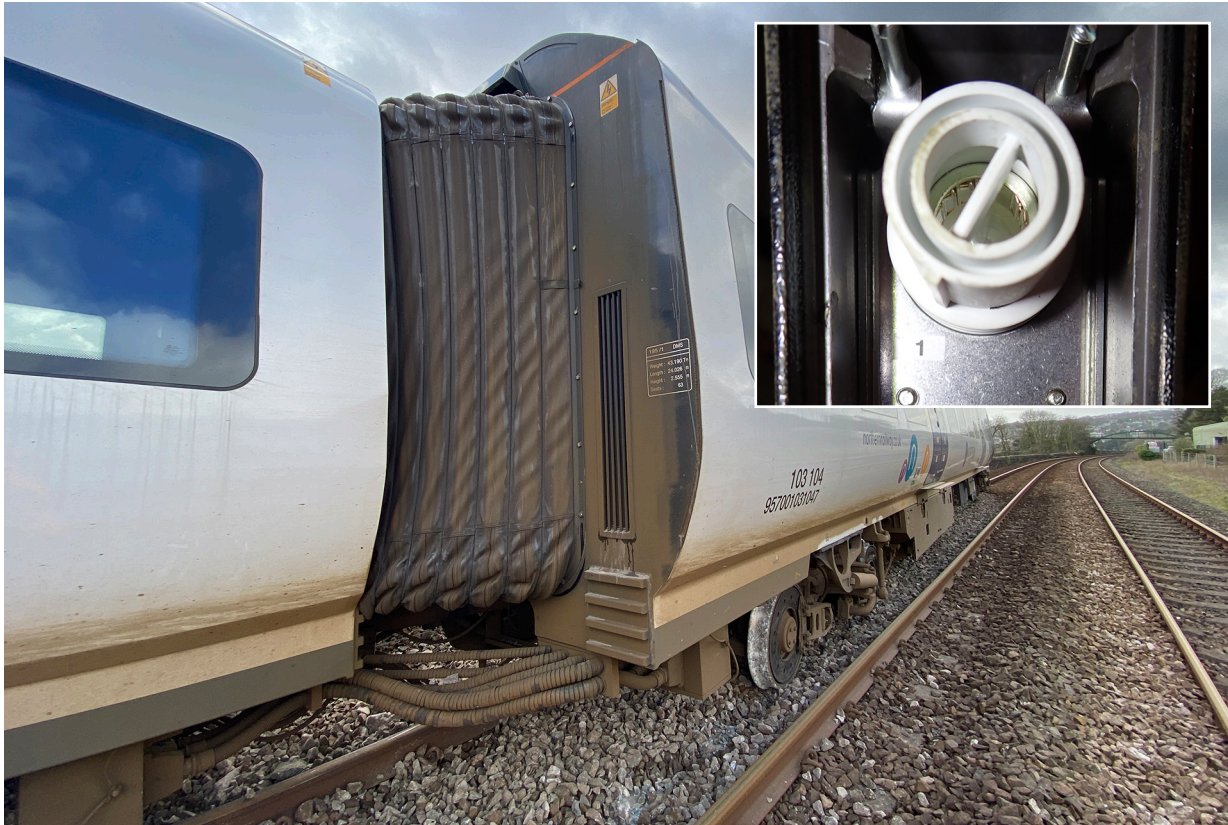
Figure 16: The power transfer cable stretched taut following the derailment (main). Damage to the internal fittings of the power cable discovered post derailment (inset).
