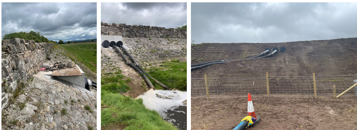
Figure 18: Railway embankment following repair by Network Rail (courtesy of Network Rail).
