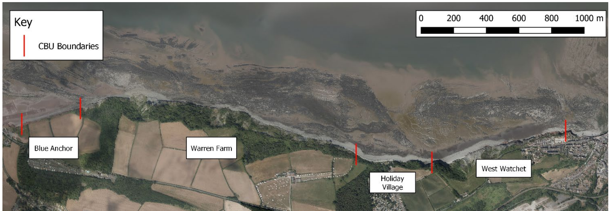
Figure 4-1: Annotated aerial photograph showing 4 cliff behavioural units (CBU) boundaries (red lines) along the coast starting at Blue Anchor along to Warren Farm, then Holiday village and ending at West Watchet.
