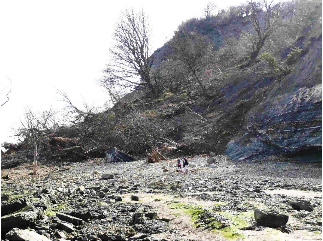
Figure 4-5: Photograph showing the Warren Farm complex landslide
