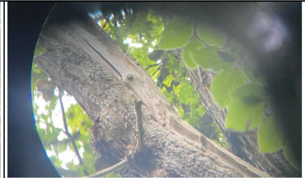
Figure 9: T1 bark decay and cracks
