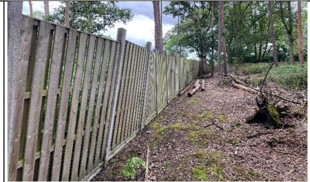
Figure 3: fencing enclosing the site
