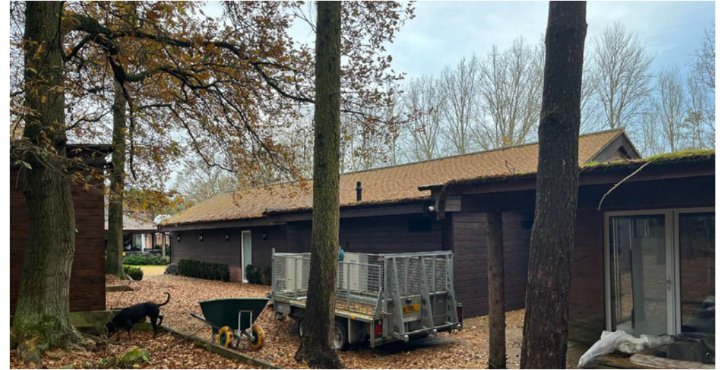
Pool House & Garage to the north of the site
