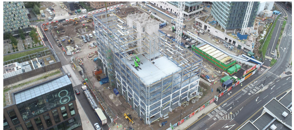
Building works progress with steel works now several floors tall.
