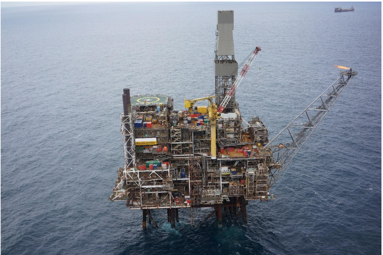
Figure 1.5.3: ANP view on east face
