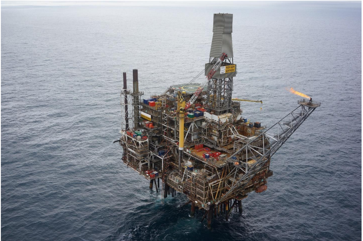
Figure 1.5.4: ANP view on north-east corner
