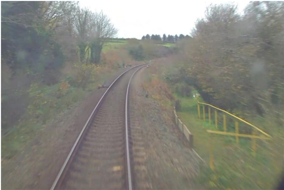
Image from forward-facing CCTV taken from a different train, showing the access point in the foreground and the bridge in the background (courtesy of Network Rail).
