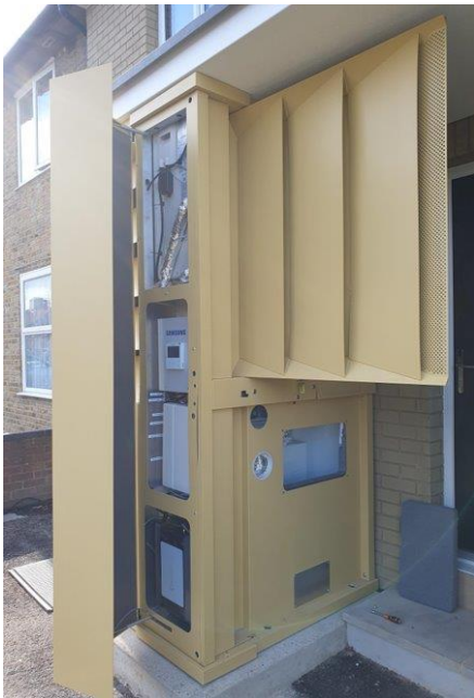
FIGURE 11 INSIDE MONODRAUGHT'S HOMEZERO MODULE
