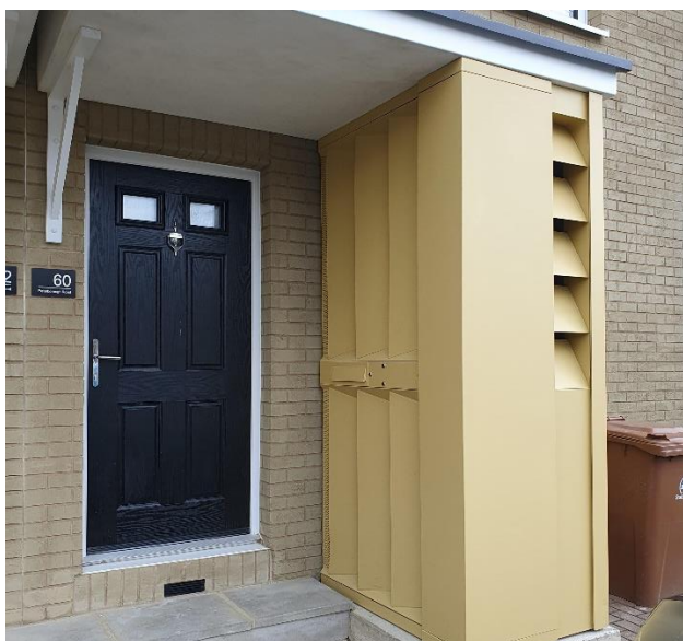
FIGURE 10 MONODRAUGHT MODULE INSTALLED ON FINISHED HOME IN SUTTON
