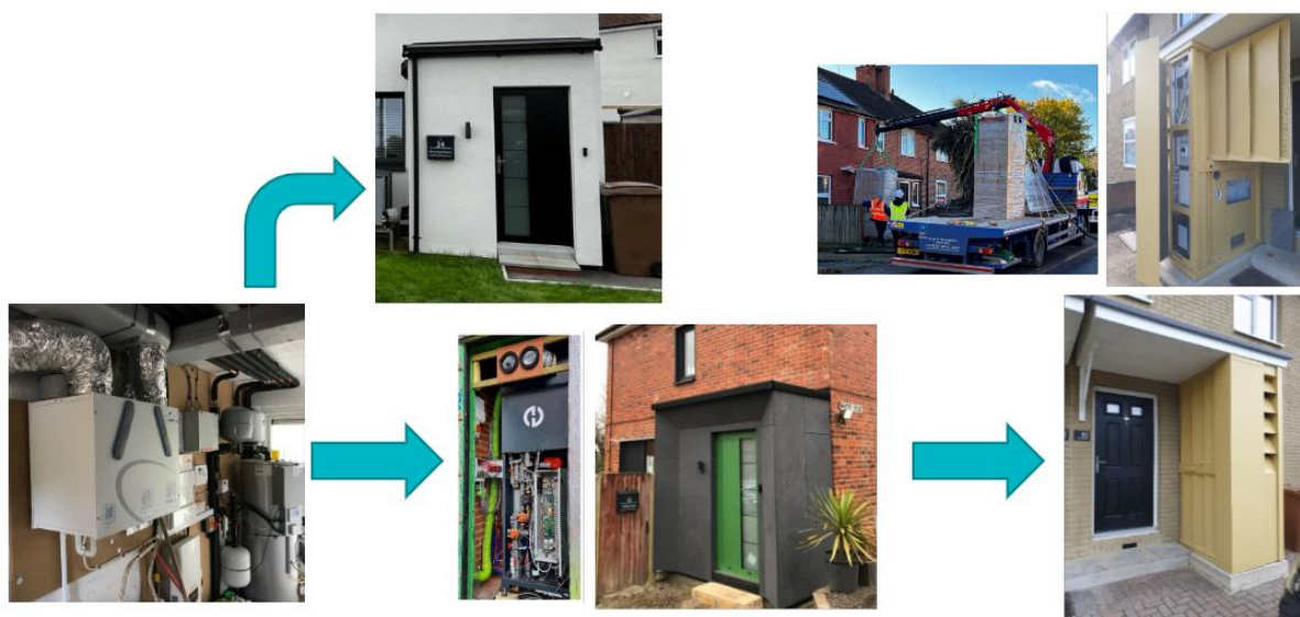
FIGURE 8 THE EVOLUTION OF ENERGY MODULES ON THE PROJECT - FROM INTERNAL ENERGY SERVICES TO INNOVATIVE PORCH PODS
