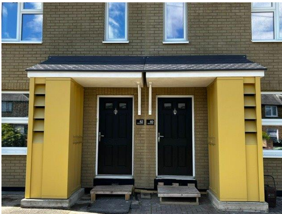
FIGURE 2 MONODRAUGHT 'HOMEZERO' ENERGY MODULES (WORKS STILL IN PROGRESS)
