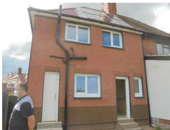
Figure 2 – Pilot property – fitted at the start with Mauer EWI system, mechanical ventilation, heating and ventilation pod, PV.
