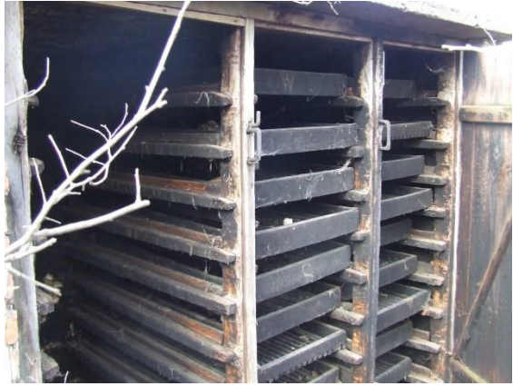
Photo 9. The oldest drying facility in Szydłów – view from the front of the drying facility to the drawers – trays
