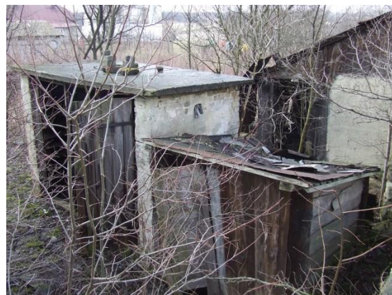
Photo 8. The oldest drying facility in Szydłów – view from above. In the lower annex there was a descent to the hearth. Wood was also stored here to dry.
