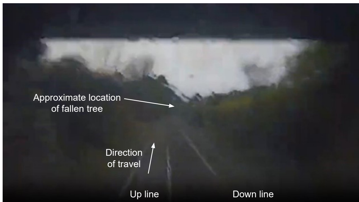
Figure 19: Image taken from train 1A37 forward-facing CCTV as it passed under the road bridge (courtesy of ScotRail with RAIB annotations).
