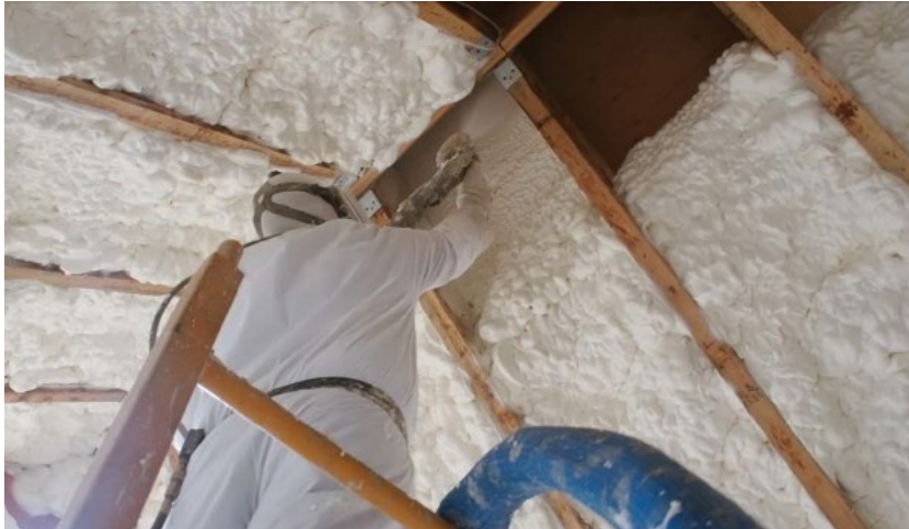
Figure 7-3: Spray foam insulation
