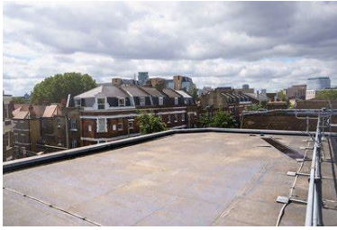
Roof regularly inspected and kept in good condition
