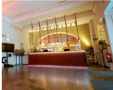
Visible wear and tear: Public spaces (e.g., bar area) have surface marks to floors and ceiling
