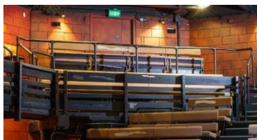
Visible wear and tear: Interior surfaces (e.g. box fronts) chipped and peeling in place
