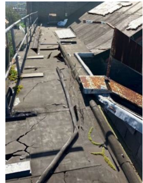
Ongoing cracks and leaks risking structural integrity of roof
