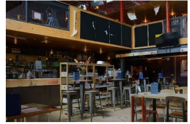
Serious damage is left unrepaired to floors, walls and ceilings
