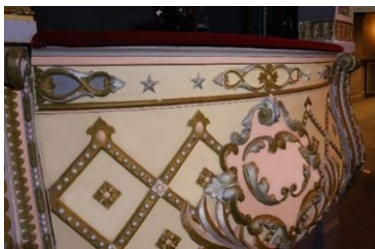
Interior surfaces (e.g. box fronts) of auditorium in good condition with minimal to no marks or damage
