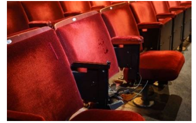
Serious damage left unrepaired: Some seats are broken and therefore unusable
