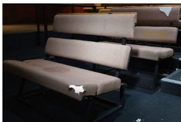
Visible wear and tear: Seats have rips and marks with some repairing
