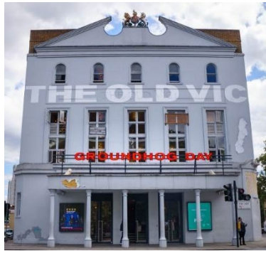
Irregular maintenance leading to paint falling away
