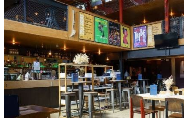
Visible wear and tear: Public spaces (e.g. bar area) have surface marks to floors and ceiling
