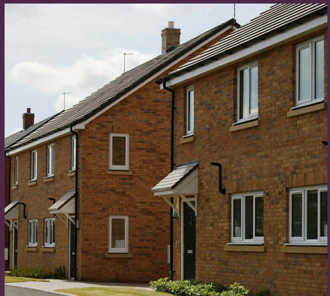
Service Family Accommodation at Beacon Barracks
