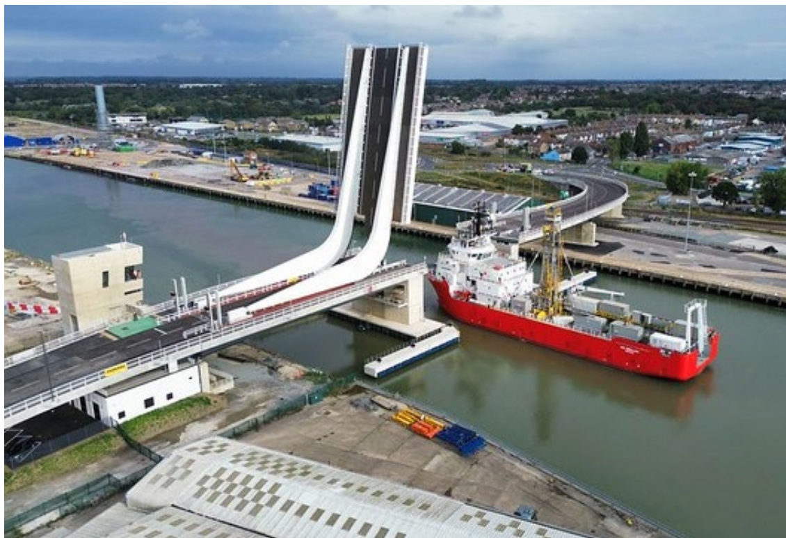
Photograph of Gull Wing – the largest rolling bascule bridge in the world. Opening day, 7 September 2024. Source: Suffolk County Council
