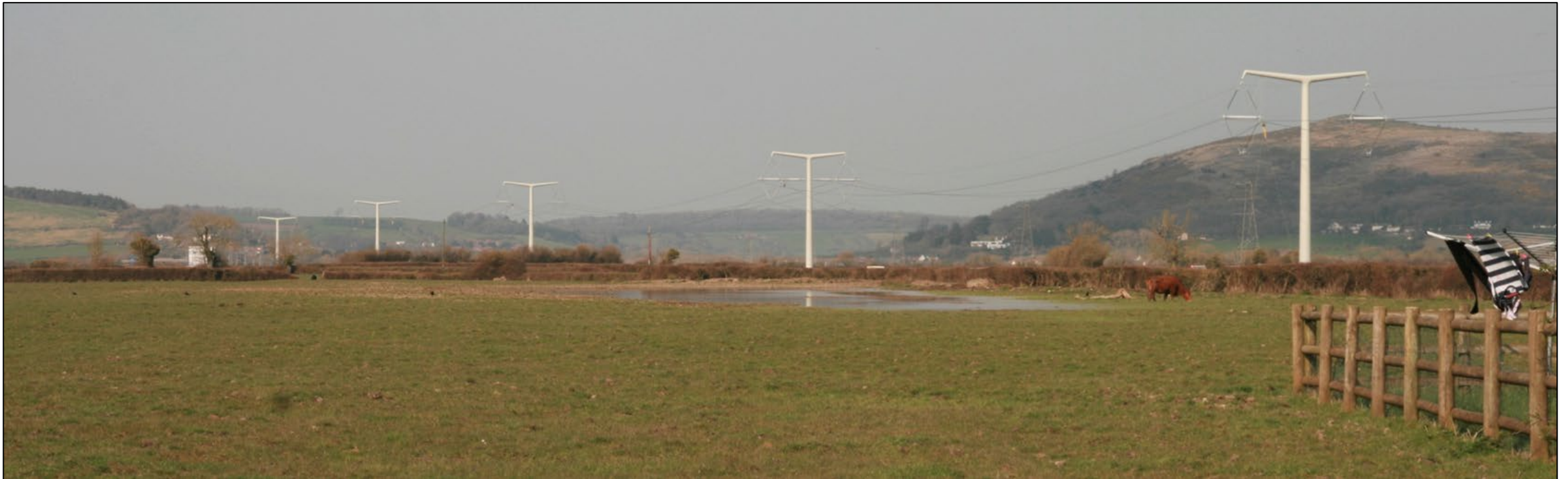
Photograph of T-pon supports across the Somerset Levels for the Hinkley Point C Connection
