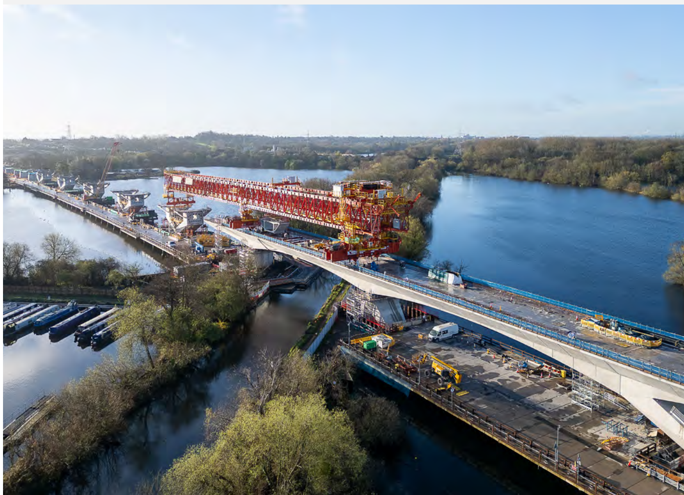
An aerial view of Colne Valley viaduct under construction. The launching girder lifts 140 tonne deck segments into place as the viaduct crosses the Grand Union Canal, which can only be conducted during periods of low wind speeds.
