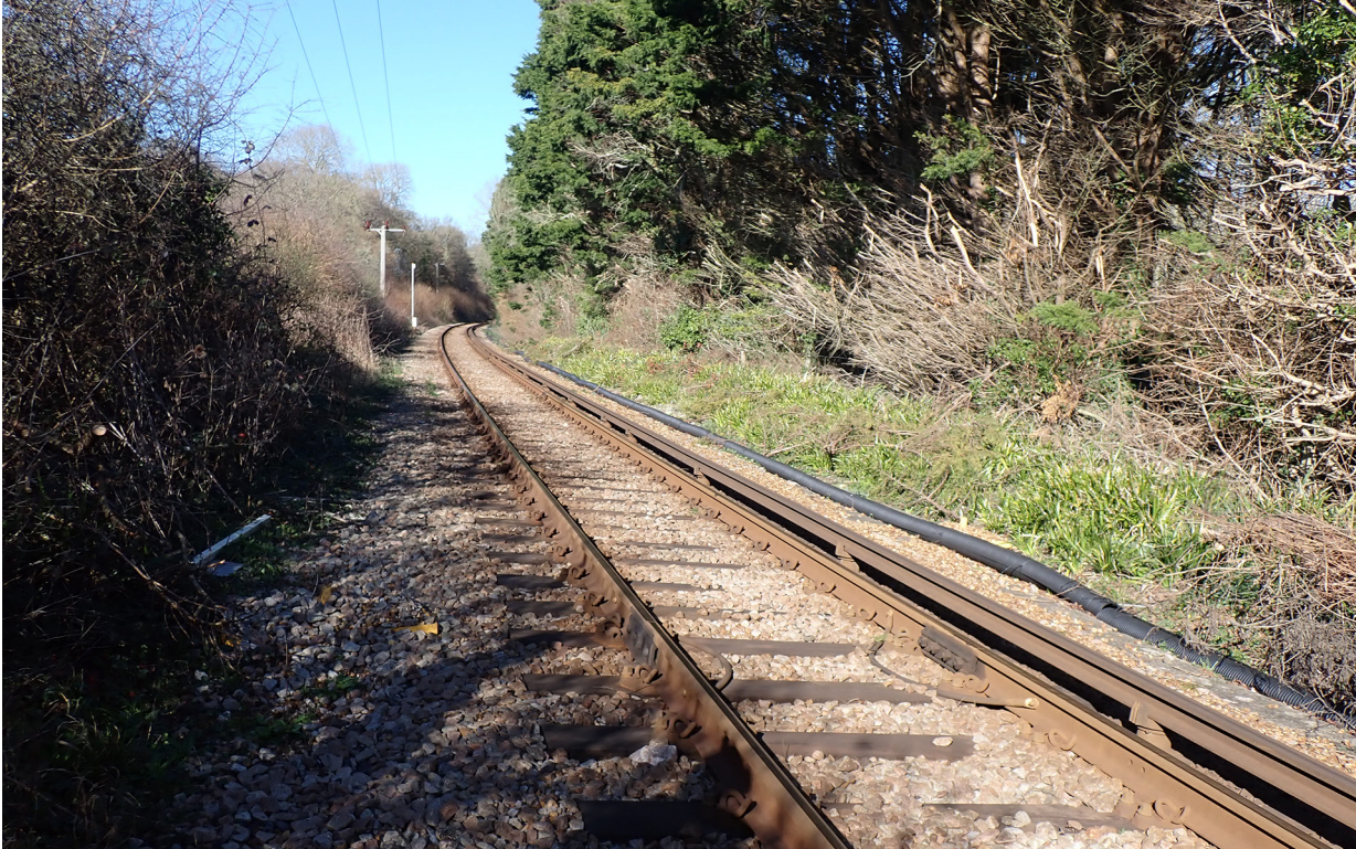
Figure 5: Location of accident looking north. The RRV approached from this direction.
