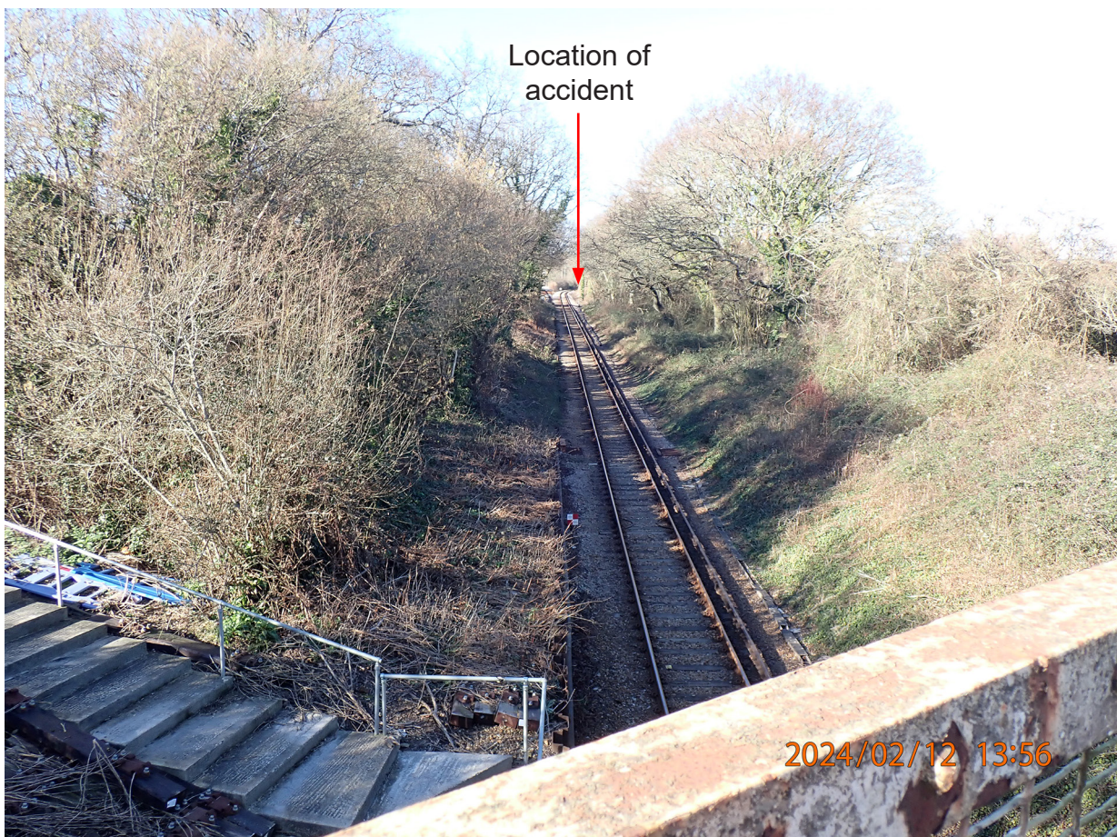
Figure 7: View from Rowborough Lane bridge looking north up the gradient towards location of accident.
