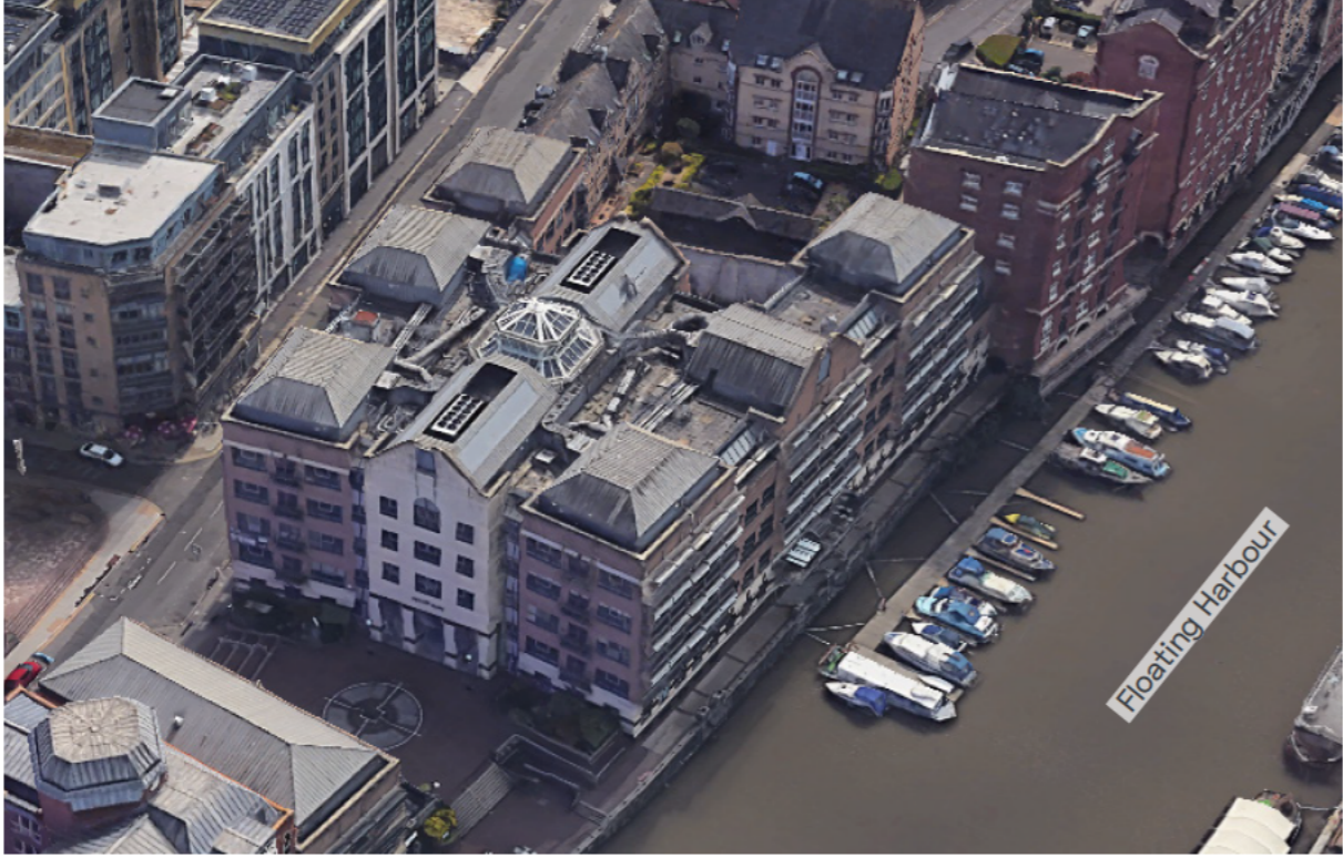
Site Aerial View - North/West façades
