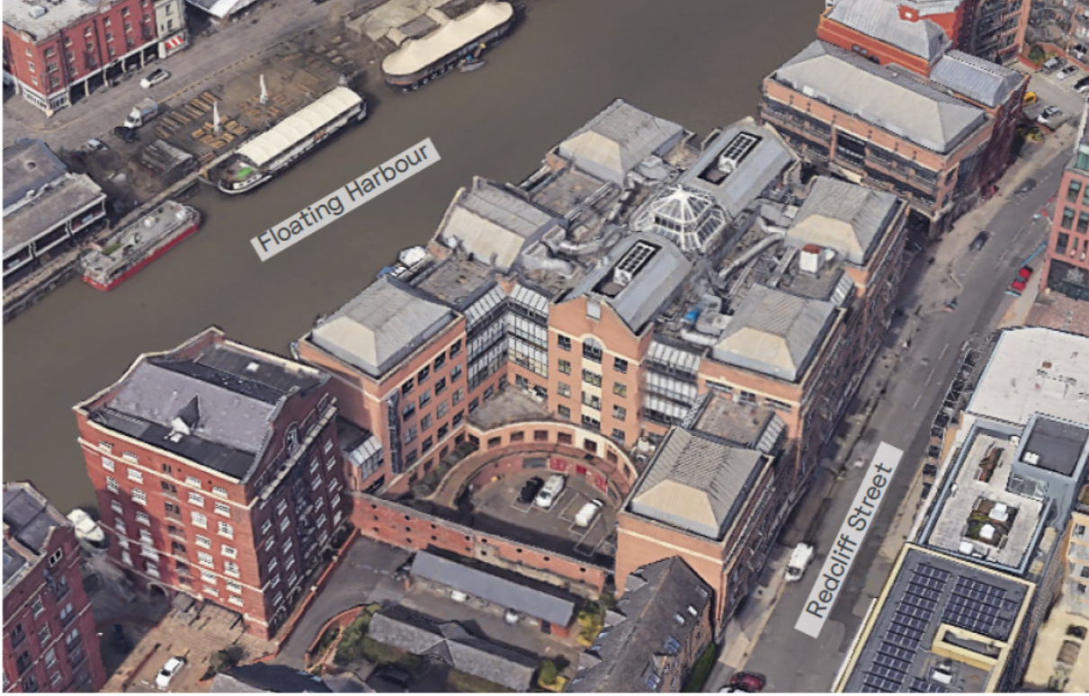
Site Aerial View - East/South façades
