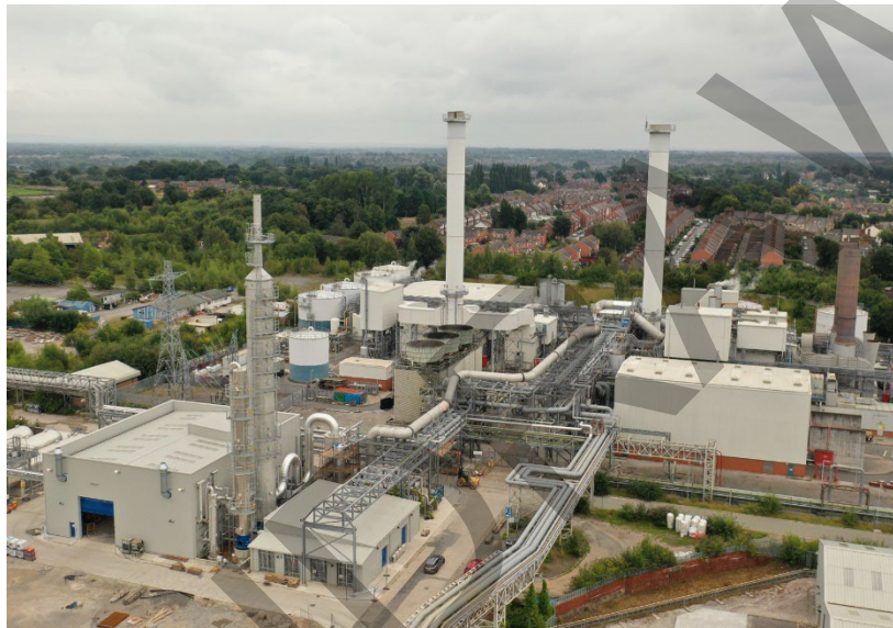
Figure 3: Tata Chemicals Europe 40,000 tCO2 CCU Facility in Northwich
