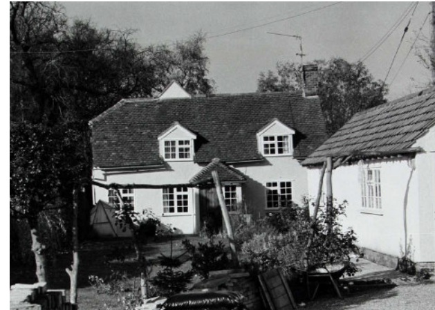
Figure 13 Beech Cottage 1975 (© Historic England)
