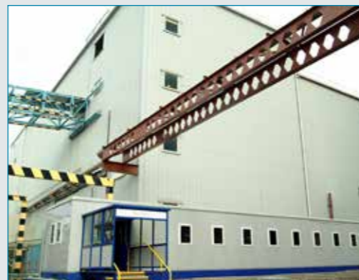
Magnox Reprocessing Plant - Sellafield
