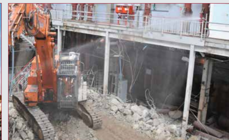
Turbine hall demolitions
