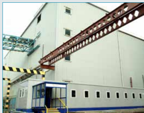
Magnox Reprocessing Plant - Sellafield
