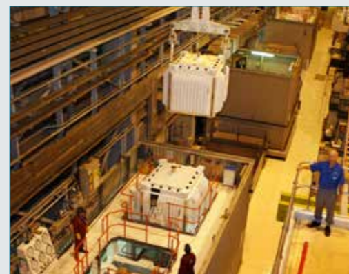
Fuel Handling Plant - Sellafield
