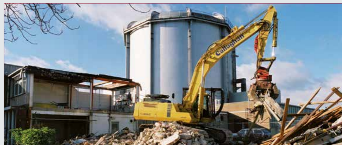
Demolition work at Harwell
