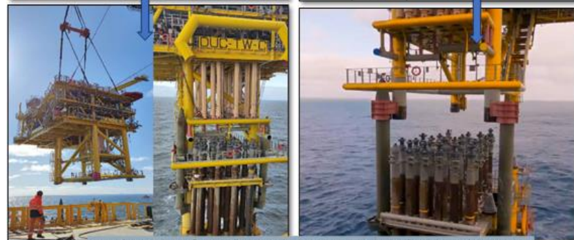
Figure 17.2: New topsides transportation and installation
