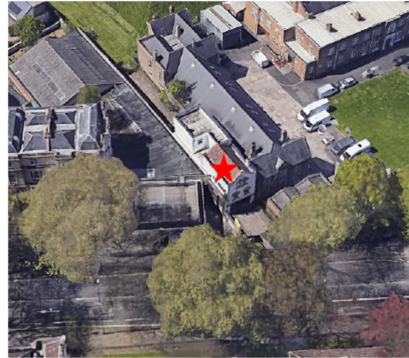
Figure 1. The site location at the west side of Whiteladies Road.
