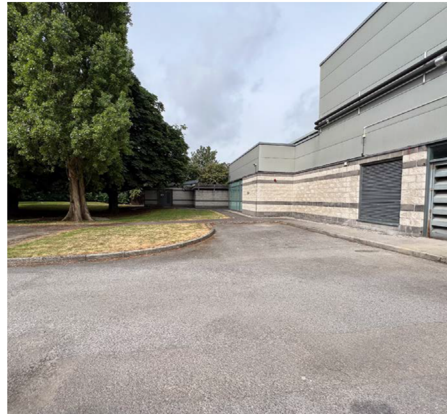
Fig. 6 Photo 2: Existing Elevation
