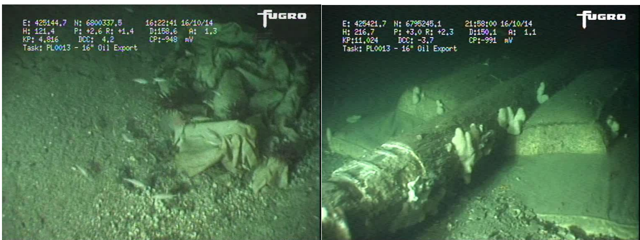
Figure 3.5.1: Examples of grout mattresses used for remediation (2014)
