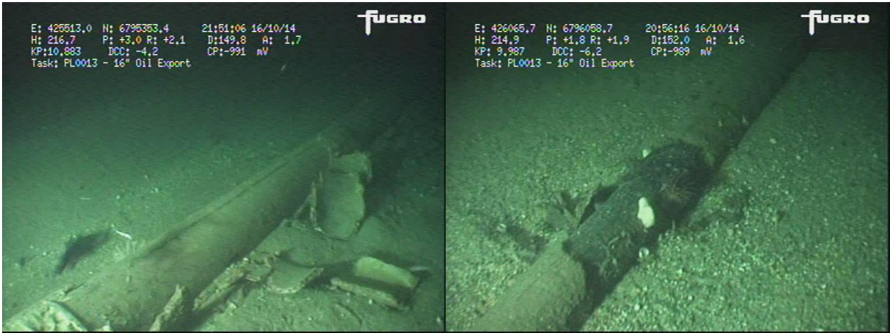
Figure 4.2.1: PL13 examples of degraded CWC (2014)
