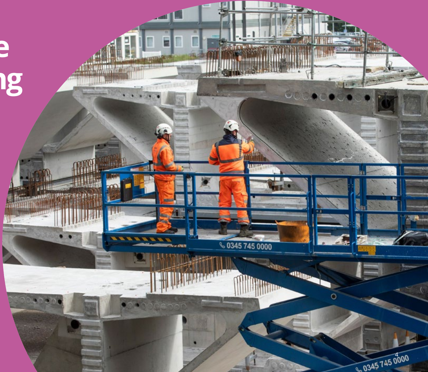
Image: Operatives preparing match cast face at the viaduct precast factory.
