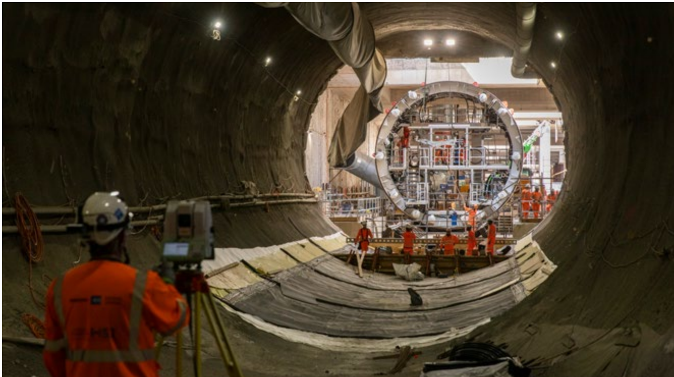
Construction works at Old Oak Common.
