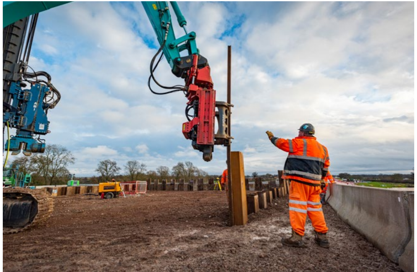
Construction works at River Blythe viaduct.
