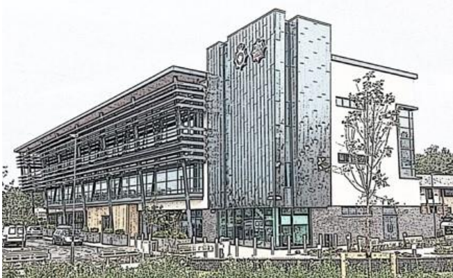
Joint-headquarters for Northamptonshire Police and Northamptonshire Fire and Rescue Service - Kettering
