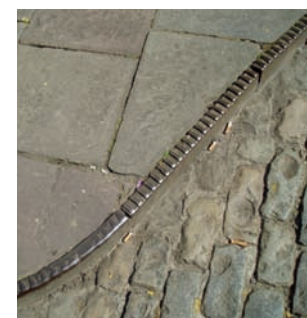
Figure 28: Examples of stone sets, iron curbs and Pennant flagstones in the Redcliffe Locality
