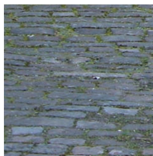
Figure 27: Pennant stone setts on Alfred Wharf
