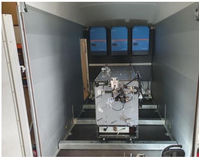
a) Fuel cell system installed in trailer
