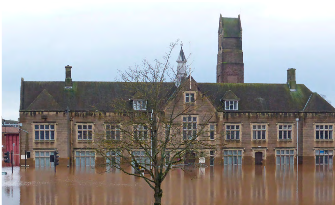
Carlisle Magistrates' Court flooding
