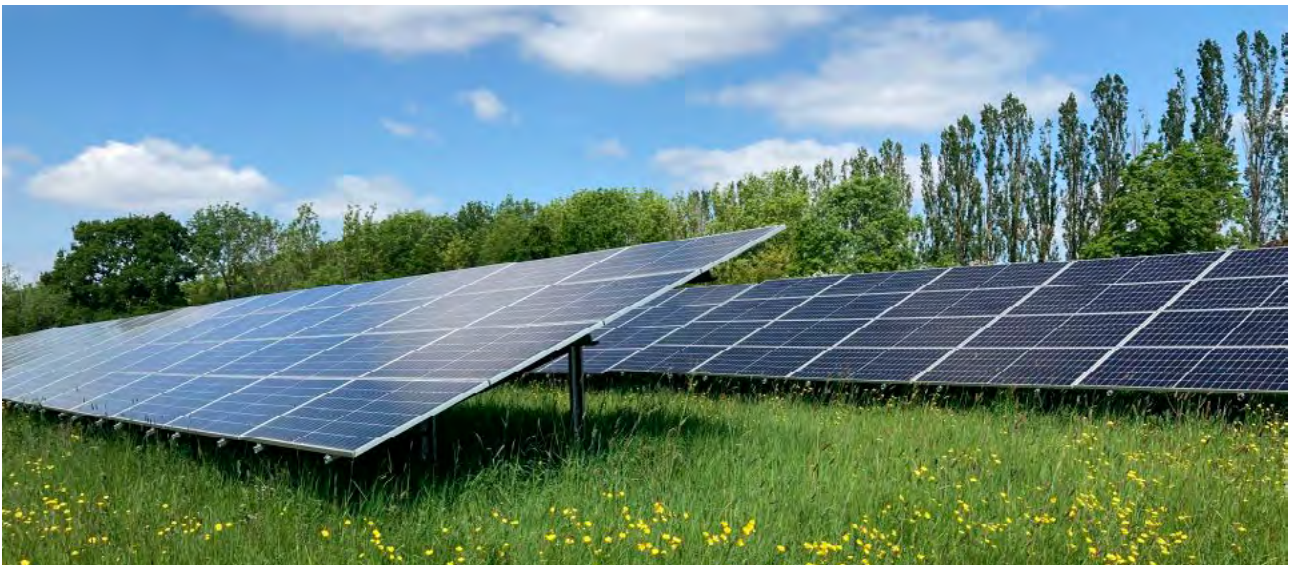
Prison Photovoltaic Array
