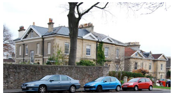
Figure 23: Nos. 4 - 10 Cotham Park, ashlar faced early Victorian villas
