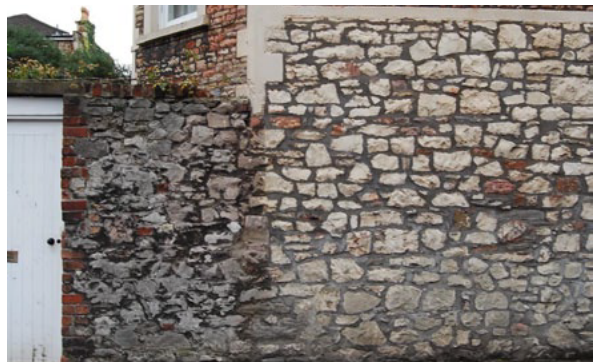
Figure 32: Stone walling materials, Kenilworth Road
