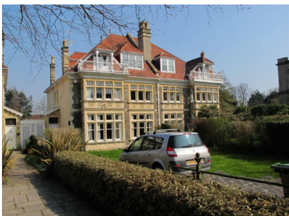
Figure 27: Nos. 18 - 20 Cotham Park
