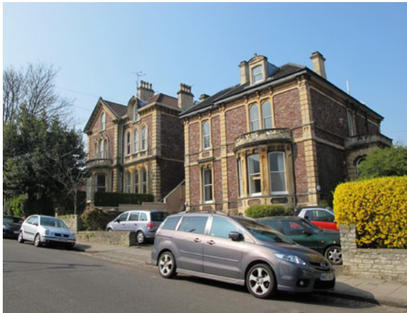
Figure 43: Red Pennant villas with limestone details, Cotham Park North
