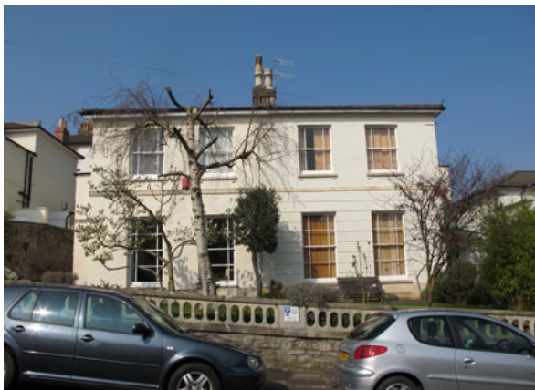
Figure 51: Typical Victorian semi, Clare Road
