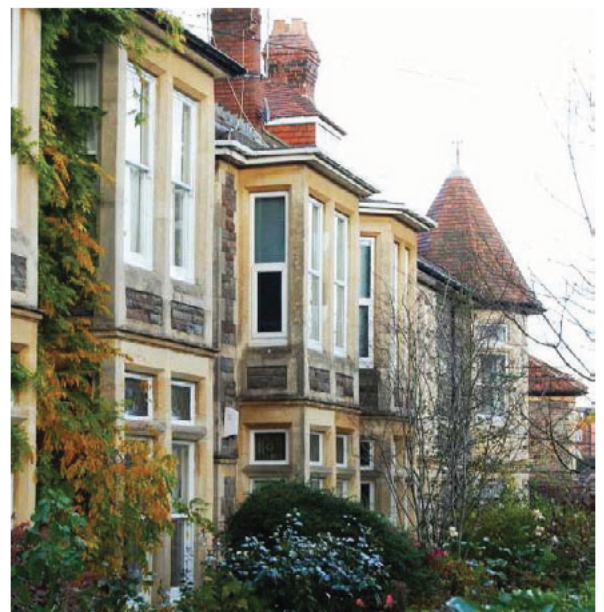
Figure 85: Canarvon Road facades
