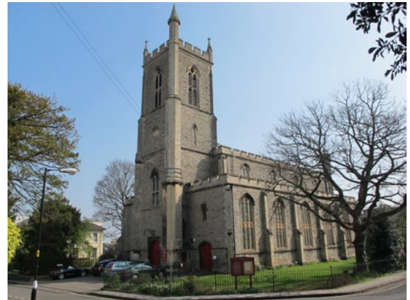
Figure 52: St Matthews Church
