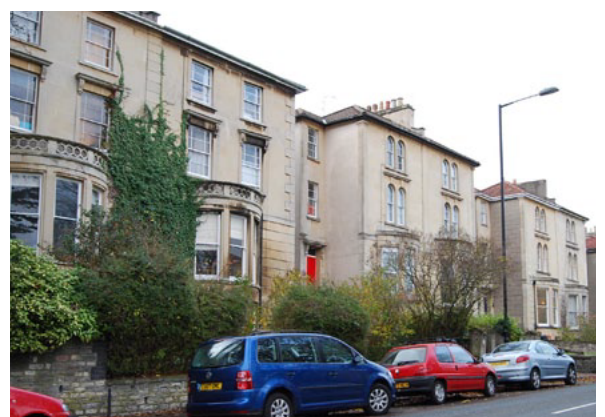
Figure 41: Cotham Grove, 3-storey over semi-basement
