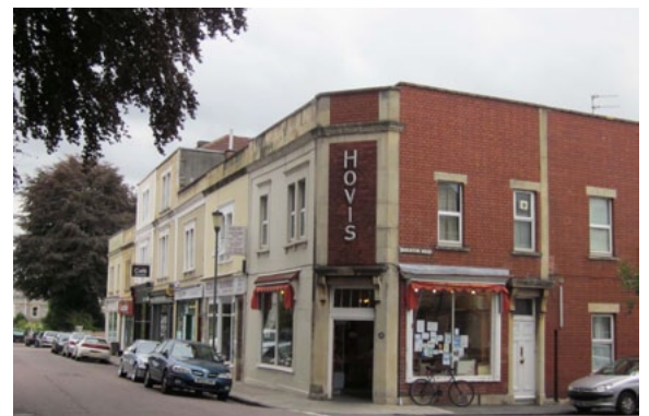
Figure 57: Nos. 1 - 30 Chandos Road
