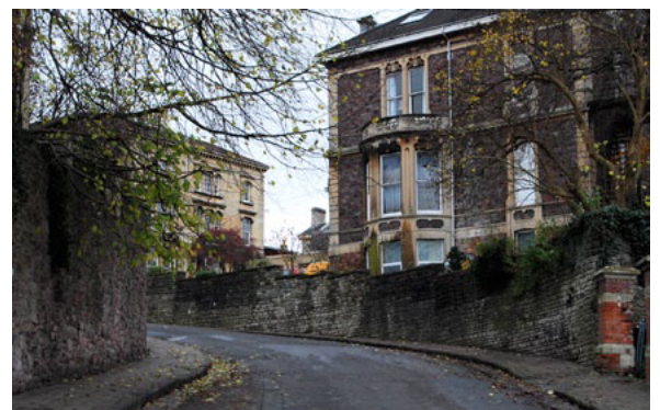
Figure 40: large boundary wall, Archfield Rd
