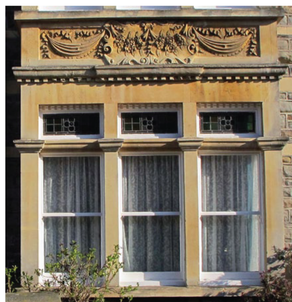
Figure 93: Late Victorian windows, Luccombe Hill
