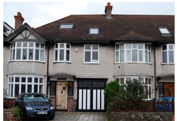
Figure 22: Inter-War houses, nos. 9 - 11 Cotham Lawn Road
