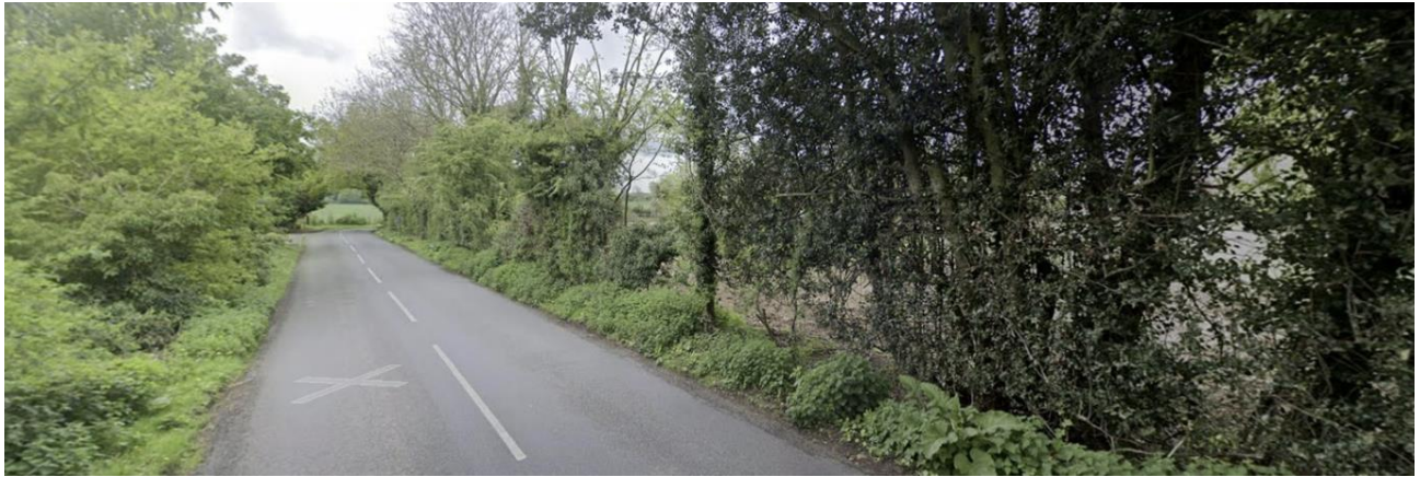
Pound Lane (no pavement, street lighting, signage)
