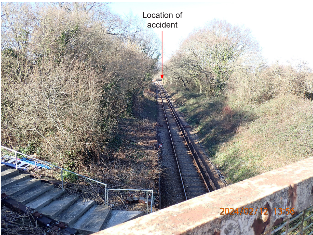
Figure 7: View from Rowborough Lane bridge looking north up the gradient towards location of accident.
