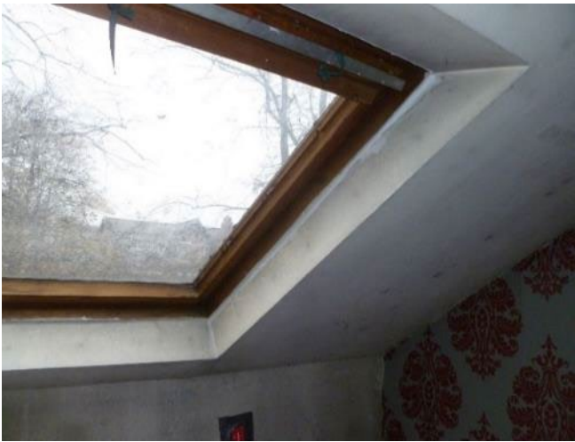
Figure 3-17 Mastic sealant applied around window frames
