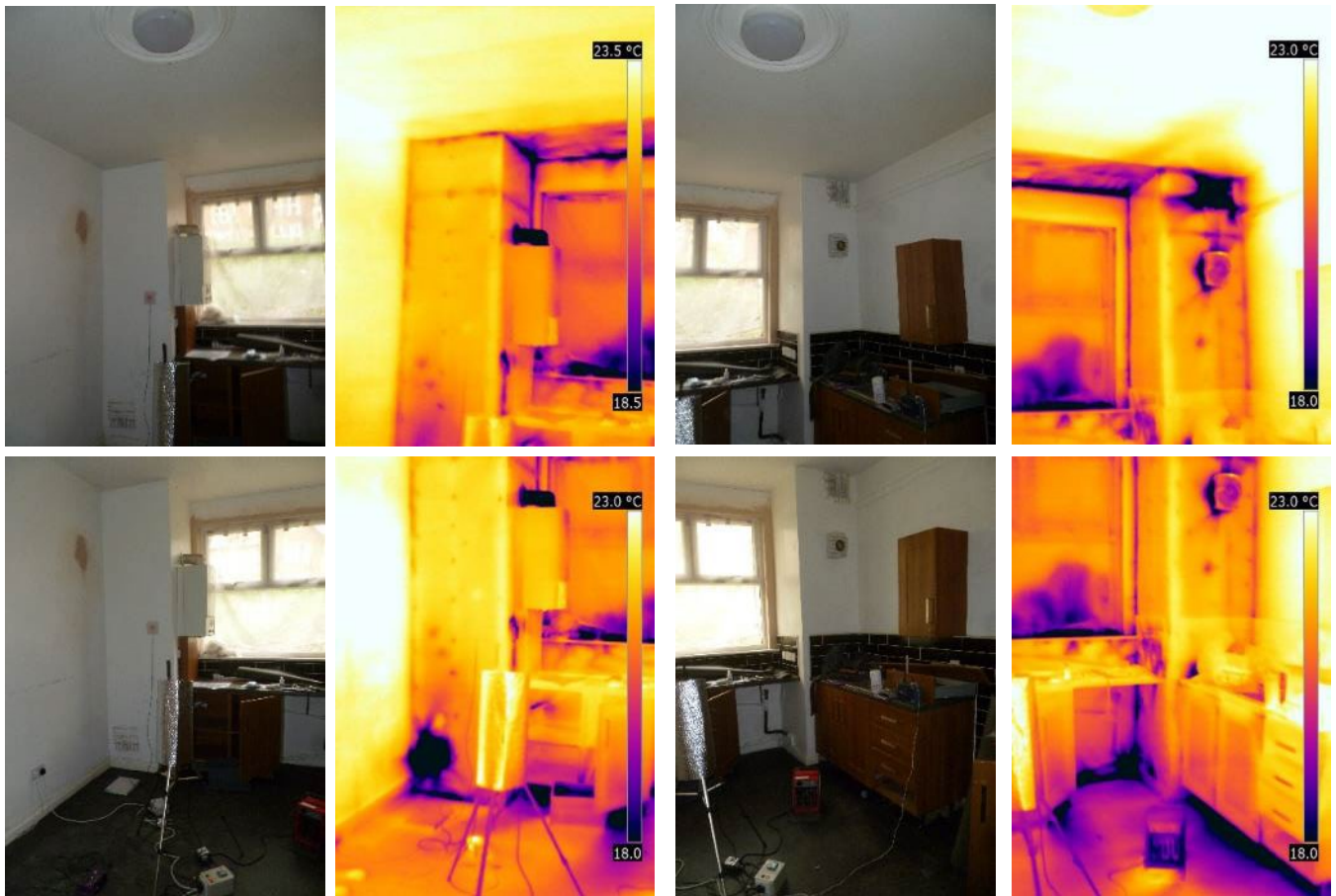
Figure 3-3 Service penetrations in the kitchen bay
