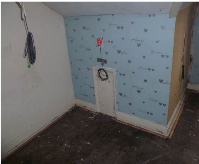
Figure 3-16 Sealed access hatches to the eaves voids
