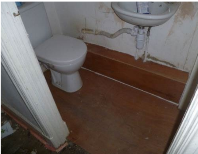
Figure 3-15 Mastic and foam fillers addressing the gaps identified in the airtightness tests
