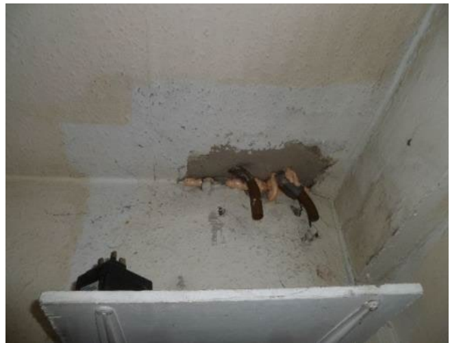
Figure 3-15 Mastic and foam fillers addressing the gaps identified in the airtightness tests
