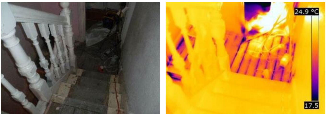
Figure 3-21 Air movement through intermediate floors in the centre of the dwelling
