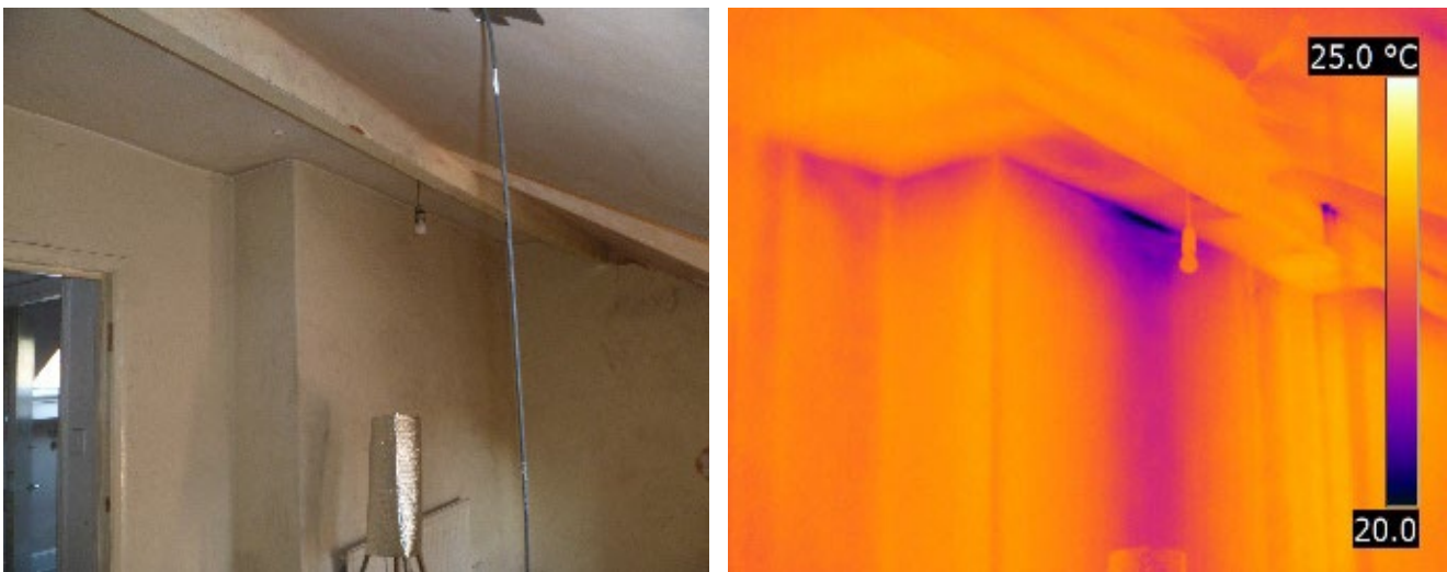
Figure 3-27 Indirect air leakage through the floor in Bedroom 1 being drawn down the chimney breast
