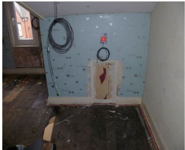
Figure 3-15 Mastic and foam fillers addressing the gaps identified in the airtightness tests
