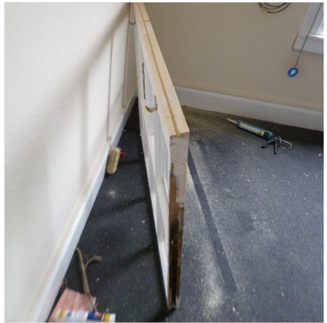
Figure 3-19 Individual sashes and beading removed, sashes repaired and beading replaced
