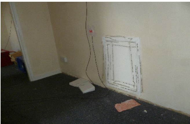
Figure 3-14 The new eaves void access hatches in 07LT, not yet fastened and draught-stripped, at the time of the post room-in-roof retrofit pressure test
