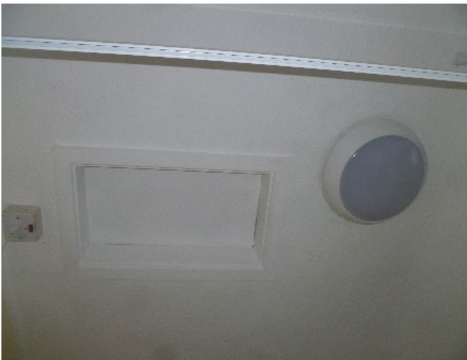
Figure 3-7 Air leakage around all loft and eaves void access hatches
