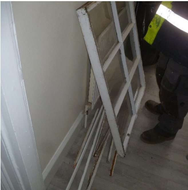
Figure 3-19 Individual sashes and beading removed, sashes repaired and beading replaced
