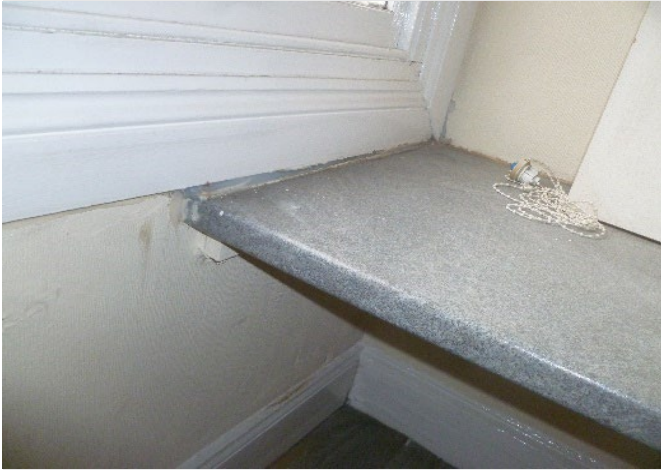
Figure 3-17 Additional sealing in the kitchen of 07LT
