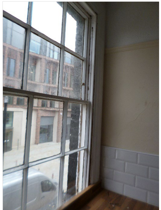
Figure 3-21 Kitchen window in 09LT removed and mechanism repaired
