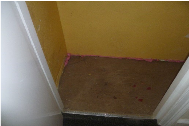
Figure 3-17 Additional sealing in the kitchen of 07LT
