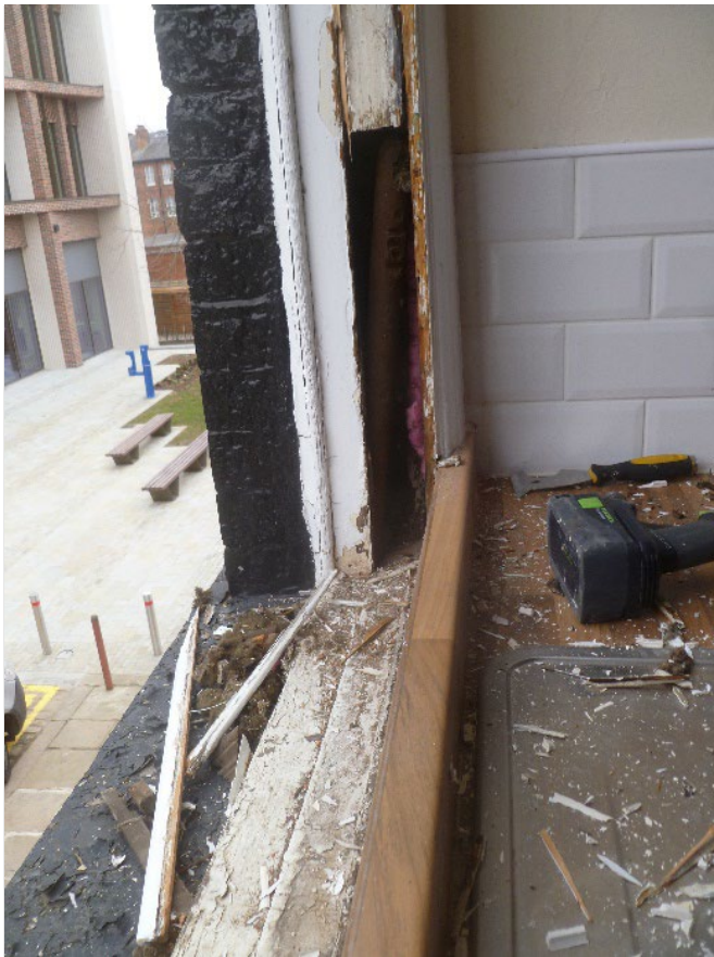
Figure 3-21 Kitchen window in 09LT removed and mechanism repaired
