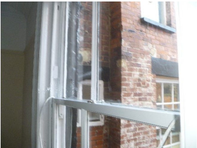
Figure 3-3 Significant air leakage at the single glazed sash windows around, and at the meeting rails between the sashes
