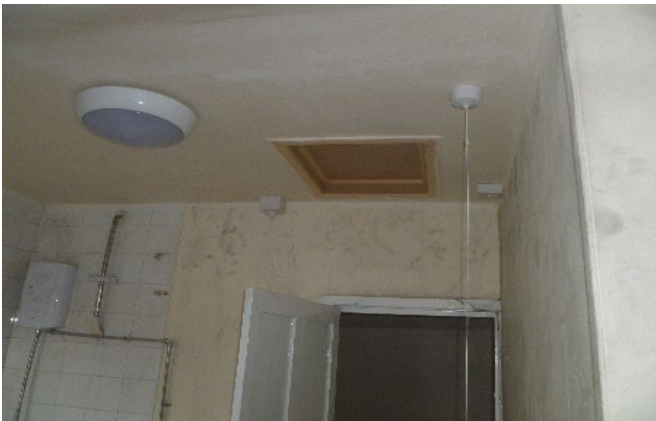
Figure 3-13 The new loft hatches, not yet draught-stripped, in 07LT at the time of the post room-in-roof retrofit pressure test
