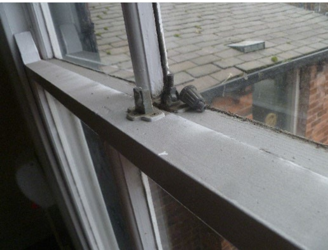
Figure 3-20 Damaged window locks replaced and new beading fitted in 07LT
