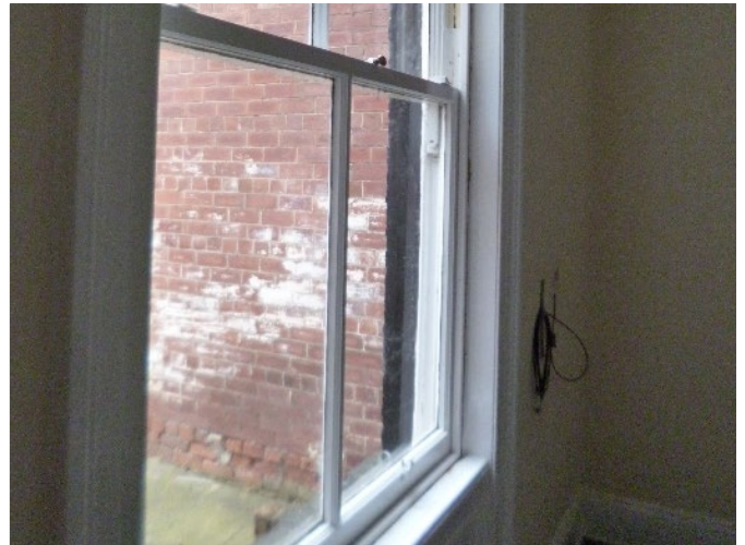
Figure 3-20 Damaged window locks replaced and new beading fitted in 07LT
