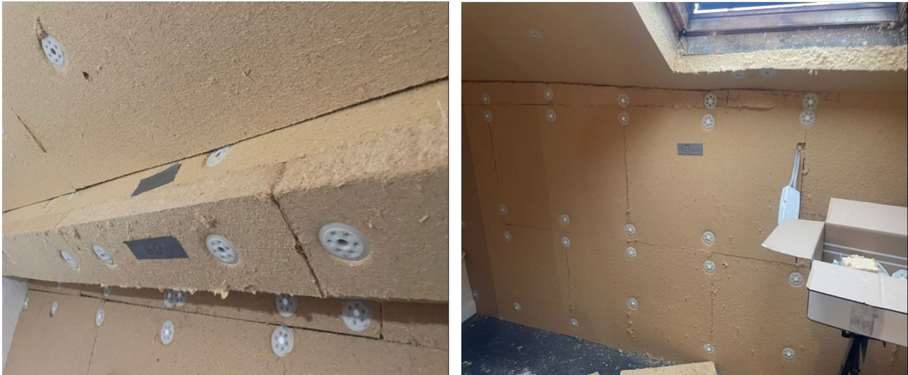
Figure 3-28 Wood fibre board installation
