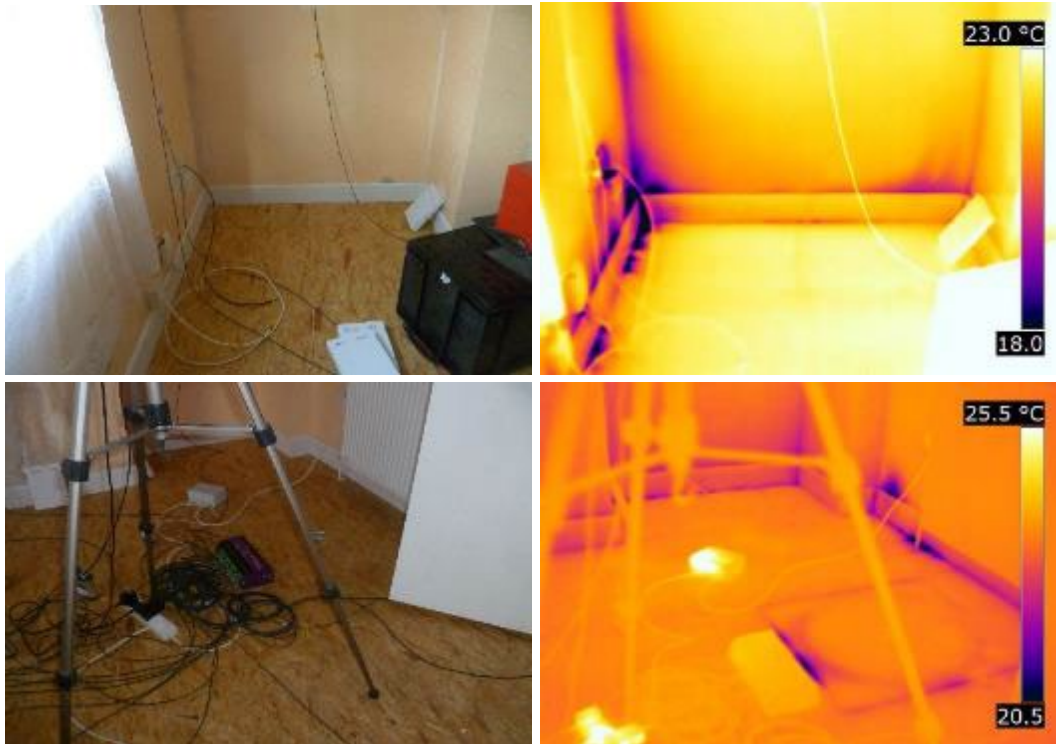
Figure 3-2 The replacement living room suspended timber ground floor under depressurisation
