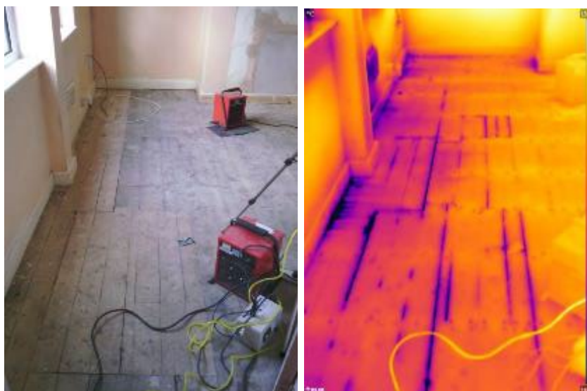
Figure 3-1 The original living room suspended timber ground floor under depressurisation
