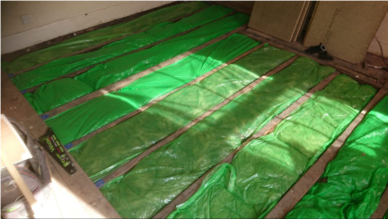
Figure 3-7 Mineral wool installed between joists
