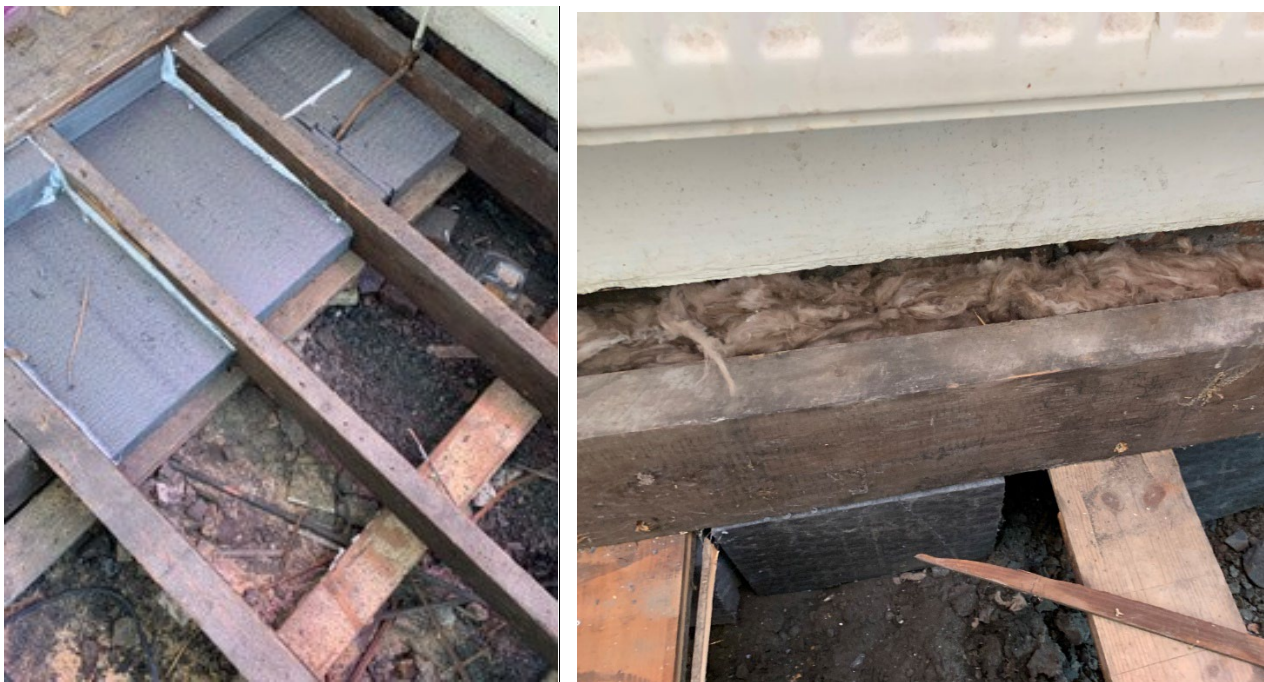
Figure 3-6 XPS installed between joists (left) mineral wool at floor perimeter (right)
